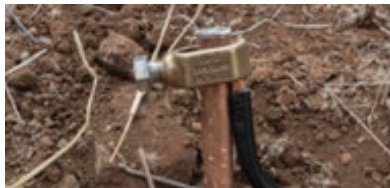
Figure 17—Earth connection
