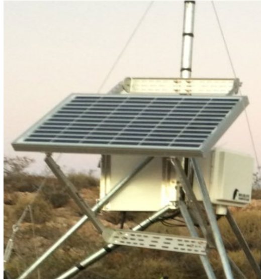
Figure 13—Solar panel mounting
