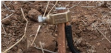
Figure 17—Earth connection
