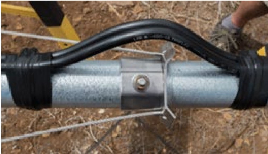
Figure 9—Coaxial cable fed around guy bracket
